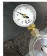
Figure 8. Checking the vacuum gauge
